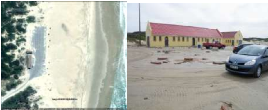
Figure 7: left) Blue Water Bay Beach parking lot located within the zone of nearshore processes, right) inundated with sand and debris after the extreme waves experienced on 1 September 2008.
