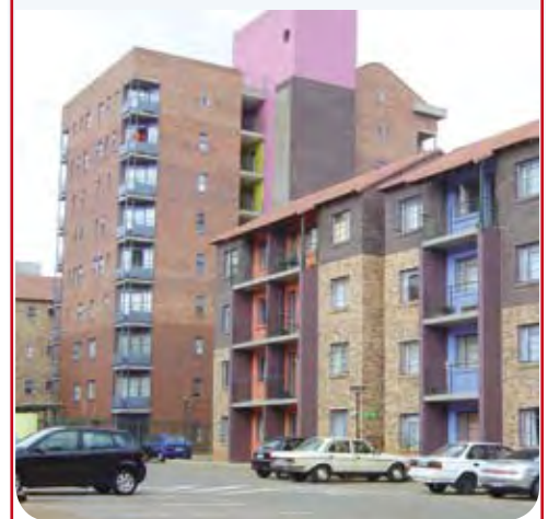
Variation in social housing blocks, Brickfields, Johannesburg
