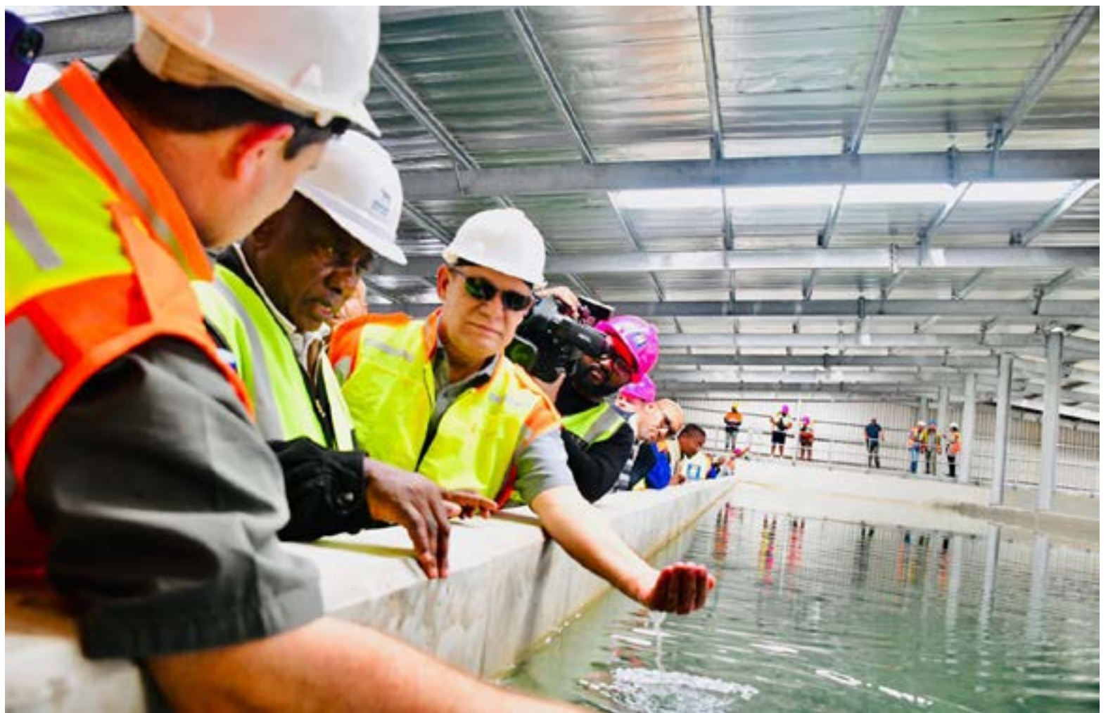
President Cyril Ramaphosa assessing the progress made with the construction of the Nooitgedagt Water Works (Phase 3) with (to his left) Barry Martin, NMBM Senior Director of Water and Sanitation
