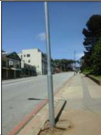
Picture 7(b): Streetlight pole replaced
