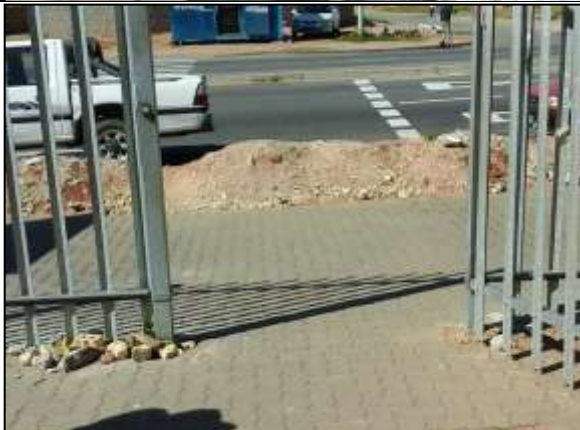
Picture 6(a): No wheelchair access at Sassa office
