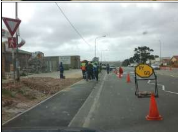
Picture 6(b): New access ramp built at entrance of Sassa office
