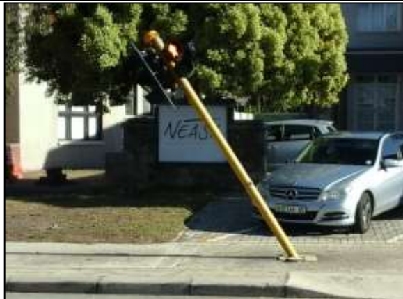
Picture 9(a): Fallen / bumped traffic light pole
