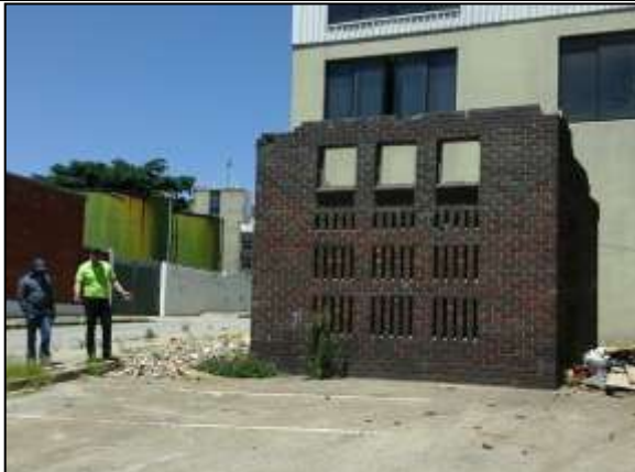
Picture 2(a): Unsightly vacant building used by vagrants
